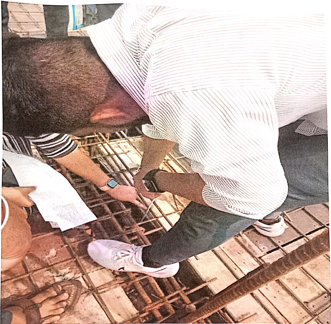
Student are checking depth of beam during visit
